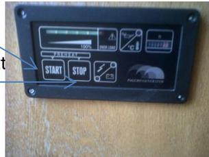
Once the generator gets going, the electric panel will make a 'click' sound after 10 seconds and the 'mains light and bulk light' will be illuminated. This means the generator is sending power successfully to the batteries. The bulk light will change to the 'absorb' light once the batteries are nearly fully charged. If neither the bulk light or absorb light illuminates after 1 minute of the generator running, call us.
